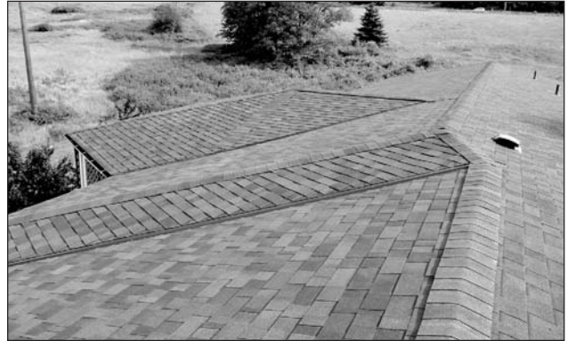
A new roof solved all leaking, rotting problems.
